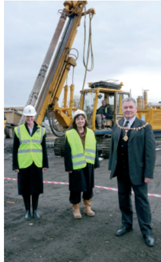
Fiona Webster, Eleanor McAllister and Provost Agnew on site at Cart Street.
