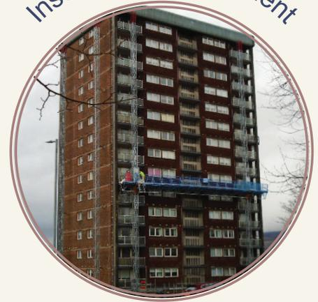
Work was carried out to upgrade the previous insulation to one that was more suitable to the buildings both in terms of heat retention, and by providing a more natural drainage system for which the cavity wall was originally designed for.
